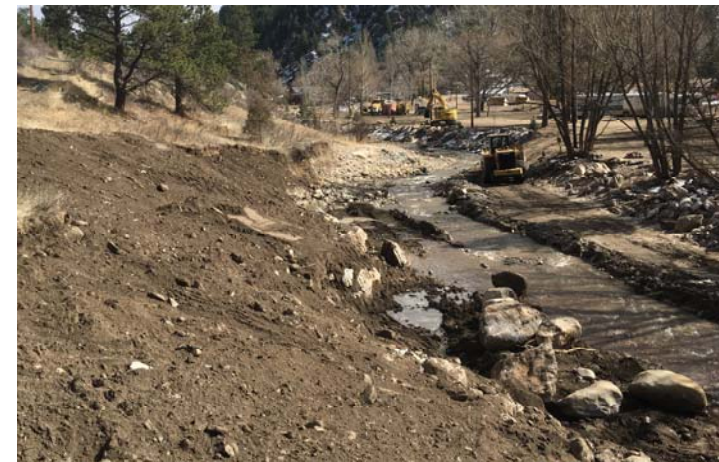
Above: Cut bank STA 15+00 to 14+00 before construction. Below: Stabilization and fill of cut bank during construction.
