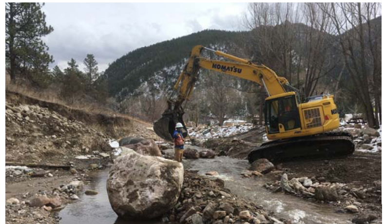
Above: Finished pool with large woody material at STA 18+00. Below: Boulder toe placement on cut slope STA 14+40.
