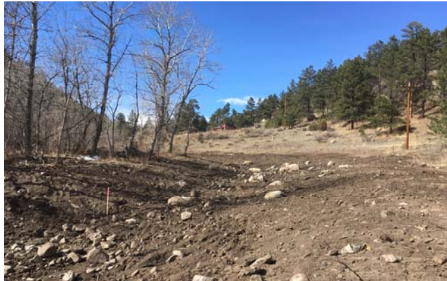
Above: Overflow channel STA 16+80. Earthwork complete, before seeding. Below: Overflow channel STA 21+60. Earthwork complete, before seeding.
