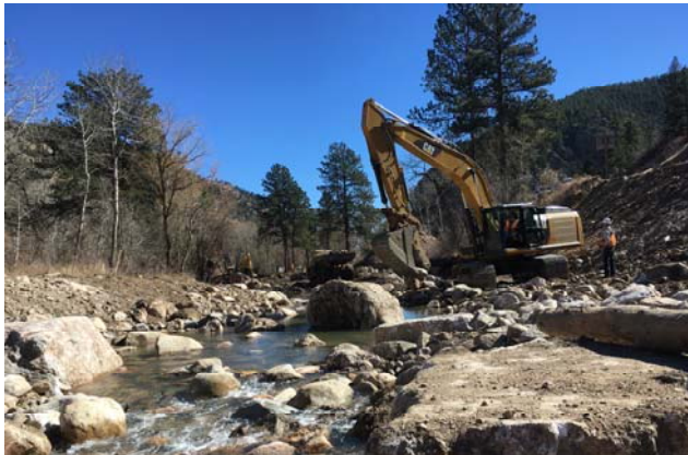
Above: Constructing boulder cascade STA 21+00 to STA 19+00 (looking downstream) Below: Finished Boulder Cascade STA 21+00 to STA 19+00 (looking upstream).
