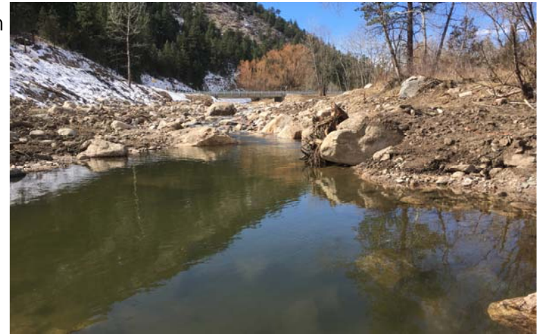
Above: Finished pool with large woody material at STA 18+00. Below: Boulder toe placement on cut slope STA 14+40.
