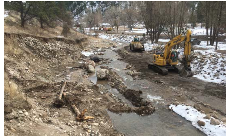
Above: Cut bank STA 15+00 to 14+00 before construction. Below: Stabilization and fill of cut bank during construction.
